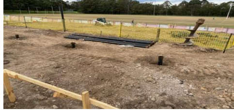
Construction starts – 13 September 2020
